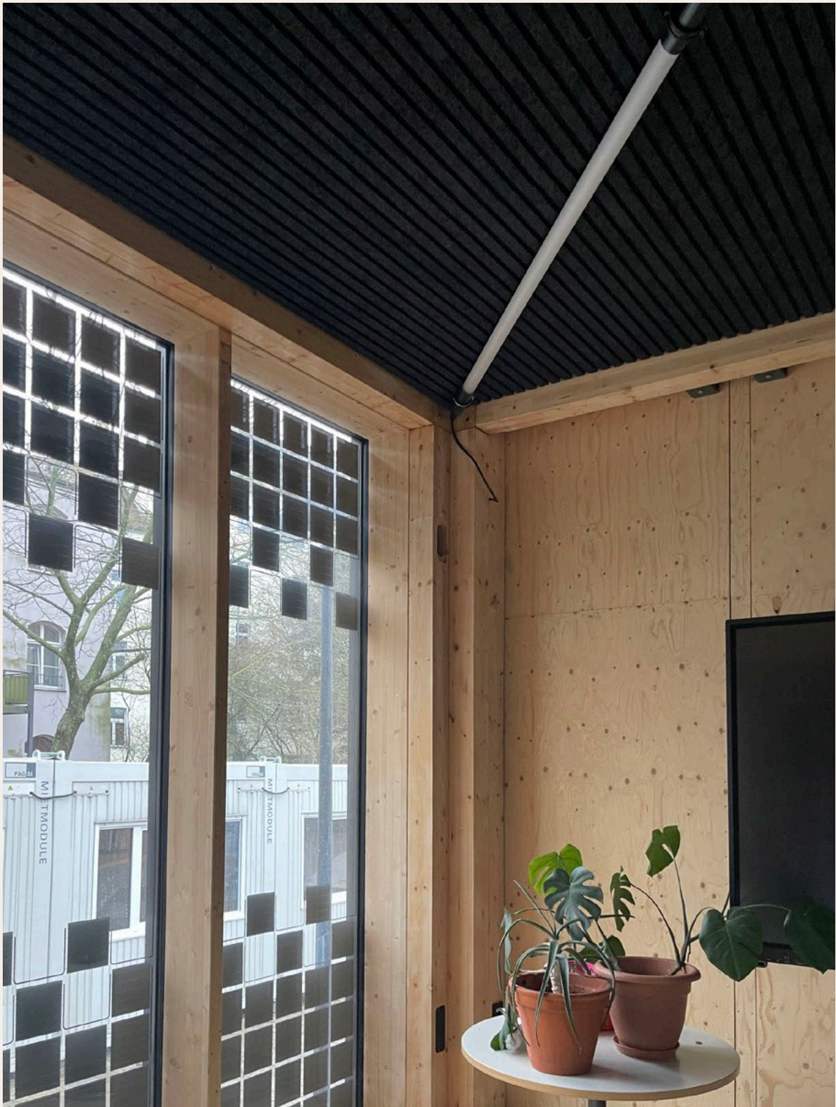
Project: Leipzig International School, Leipzig, Germany Concept Developer: Urban Beta Troldtekt products: Troldtekt acoustic panels, Troldtekt line (black 208, Cradle to Cradle Certified® at gold level)
