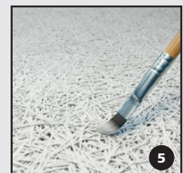
Use touch-up paint with the same colour as the panel
